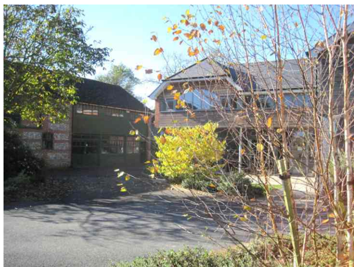
View of Project Workshops
